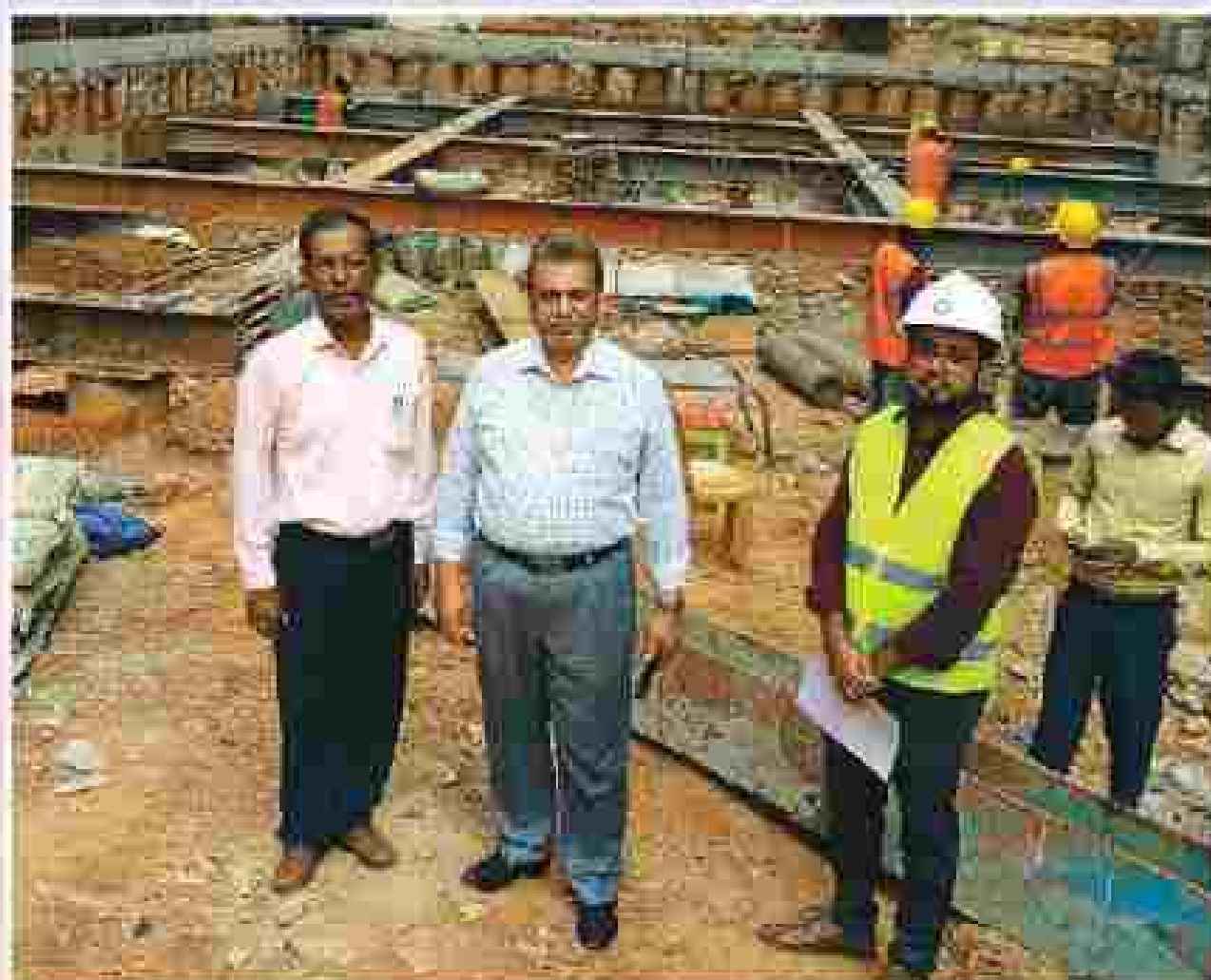
MD & CEO with the Project Manager in discussion at the Construction Site.
