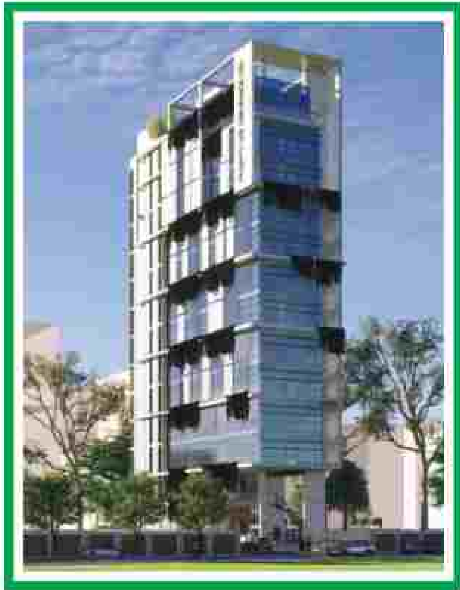
PLIPLC Head Office (Under Construction)
